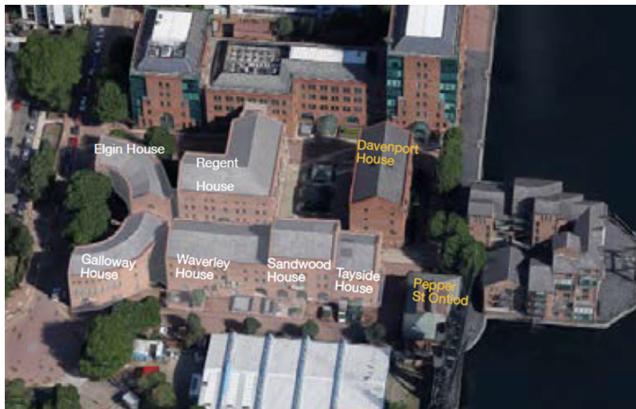
Fig.2 – Aerial View of Application Site
